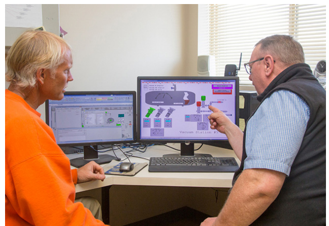
Many vacuum station operations can be monitored and adjusted from a control desk.
