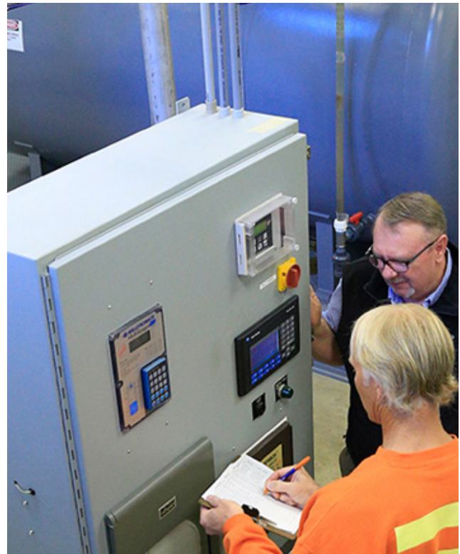
Marshall Read and Miles Beach have been instrumental in Ocean Shores’ vacuum-sewer operation for the last two decades. Here they conduct a daily vacuum station check in a clean working environment.
