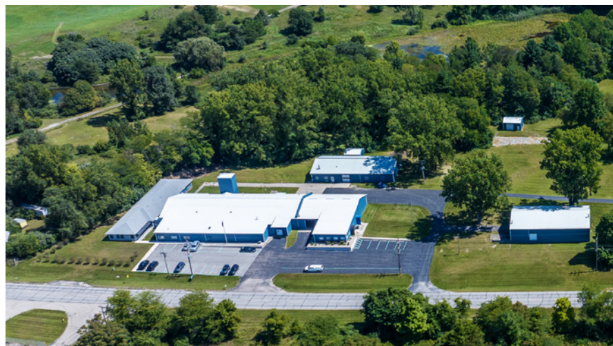
Airvac Administrative, Engineering, and Manufacturing Buildings.
