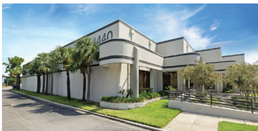
Airvac Customer Solutions Center.
